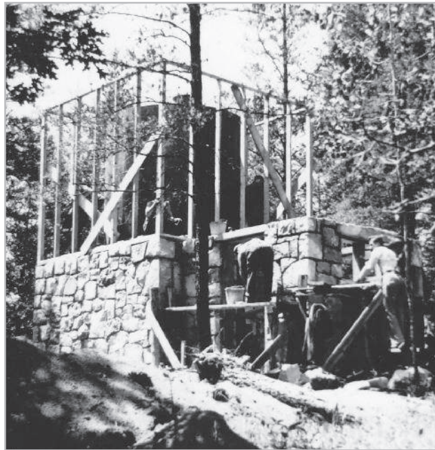
A water tower under construction at the St. Croix Recreation Demonstration Area, which is designated a National Historic Landmark, near Hinckley, Minnesota. (MN DNR)
